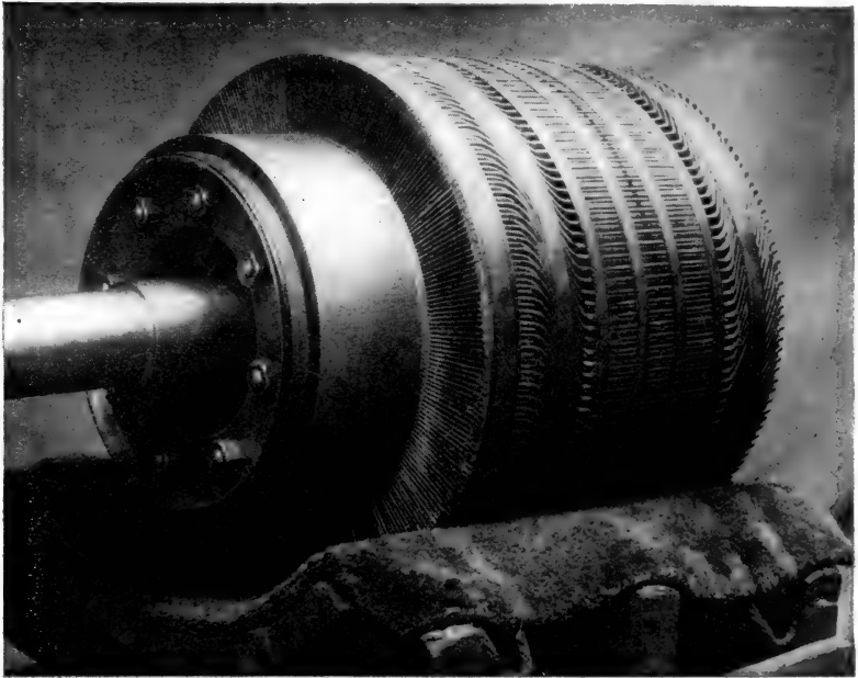
FIG. 168.—Completed Lap Wound (Multiple-circuit) Armature.
